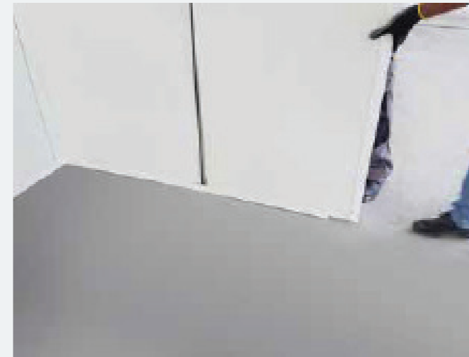
3 The panels slide into the base profiles. No technical experience is necessary for the installation of the magnetic system
