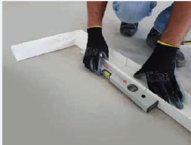
1 Build the frame of the Magnetic Ambience using profiles from the magnetic kit.
